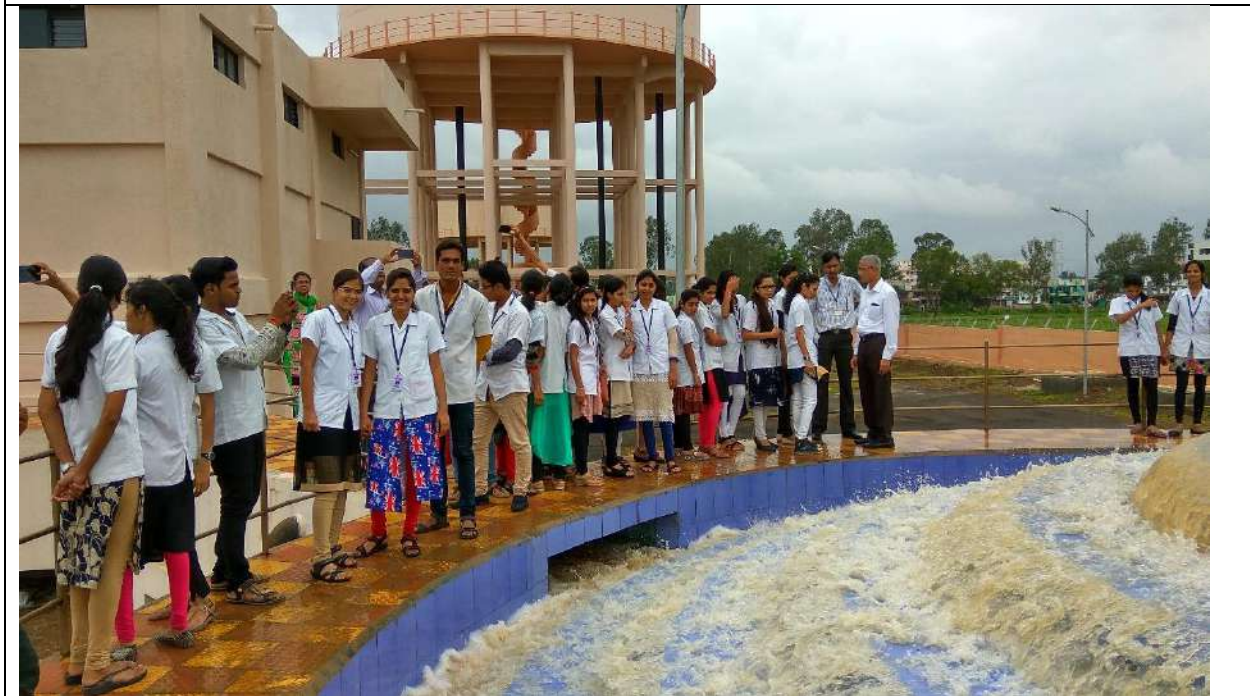
Aerator before water treatment
