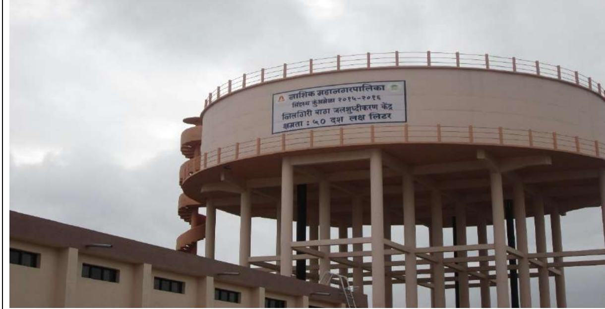
Nilgiriabaugh Water treatment plant
